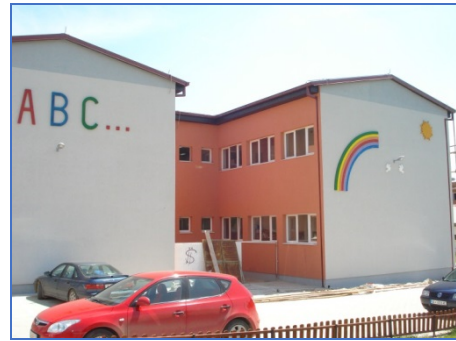
Situation after rehabilitation
