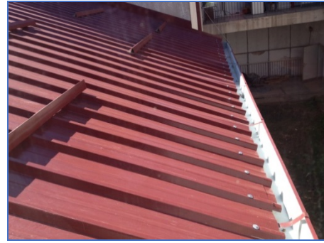
Situation after rehabilitation
